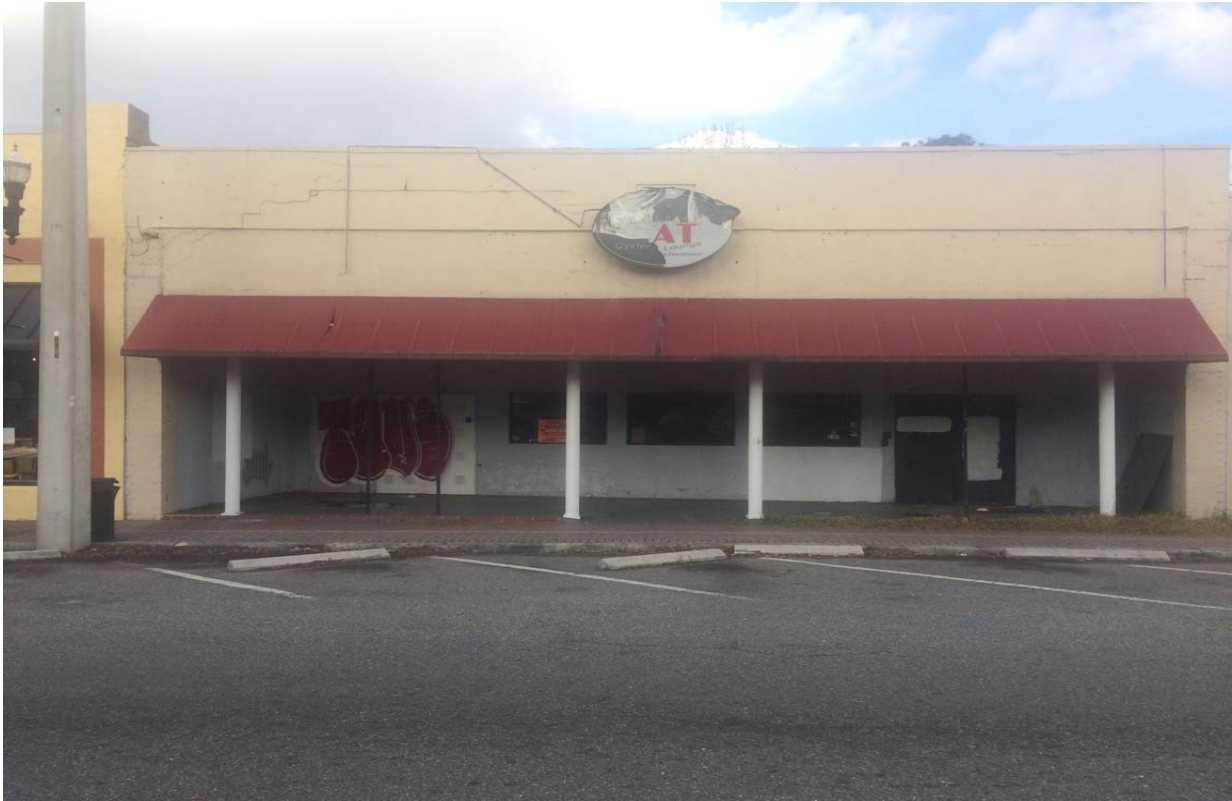
The subject site facing northeast from Edgewood Ave.
